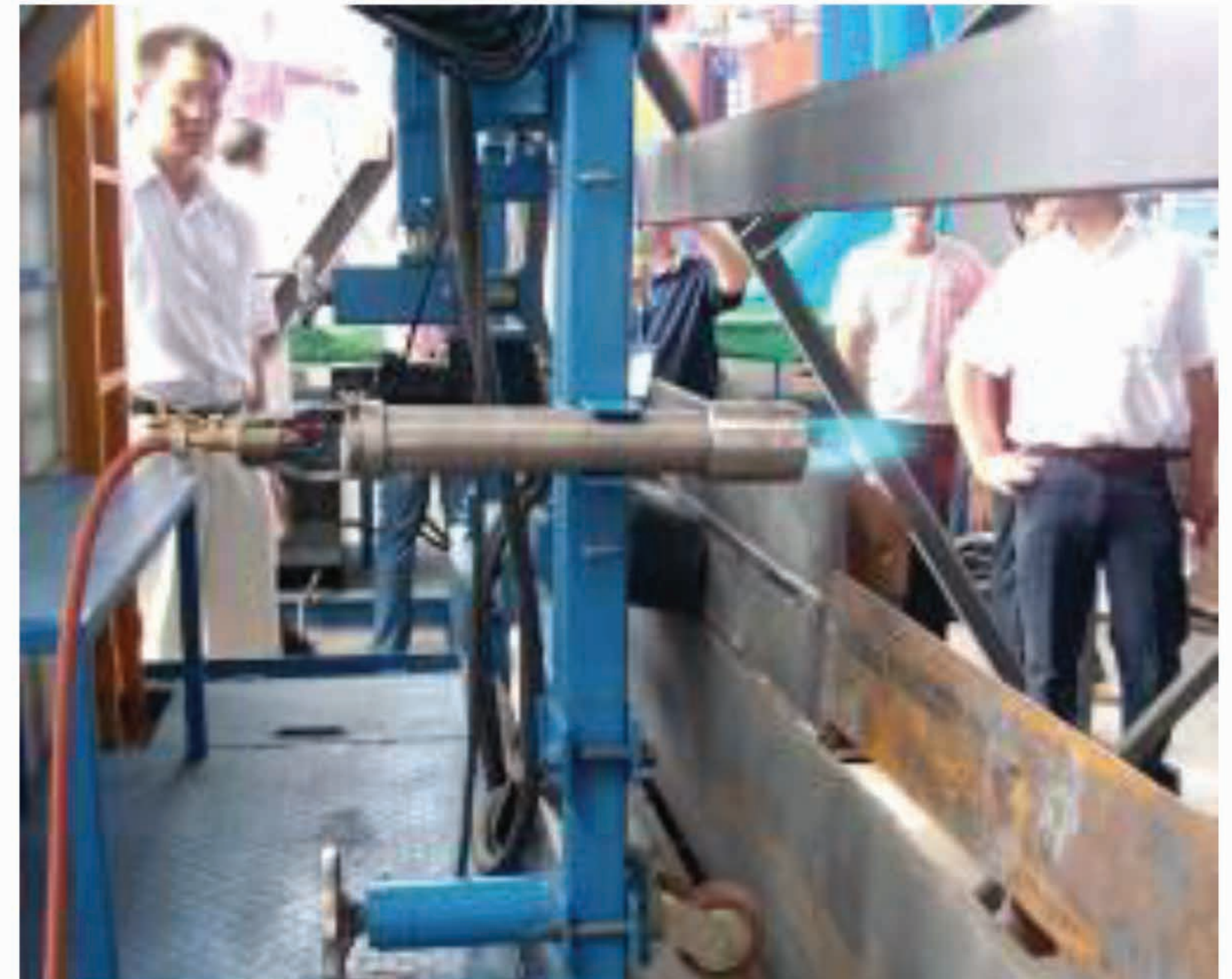
Preheating Torch for Girth Seam Welding
