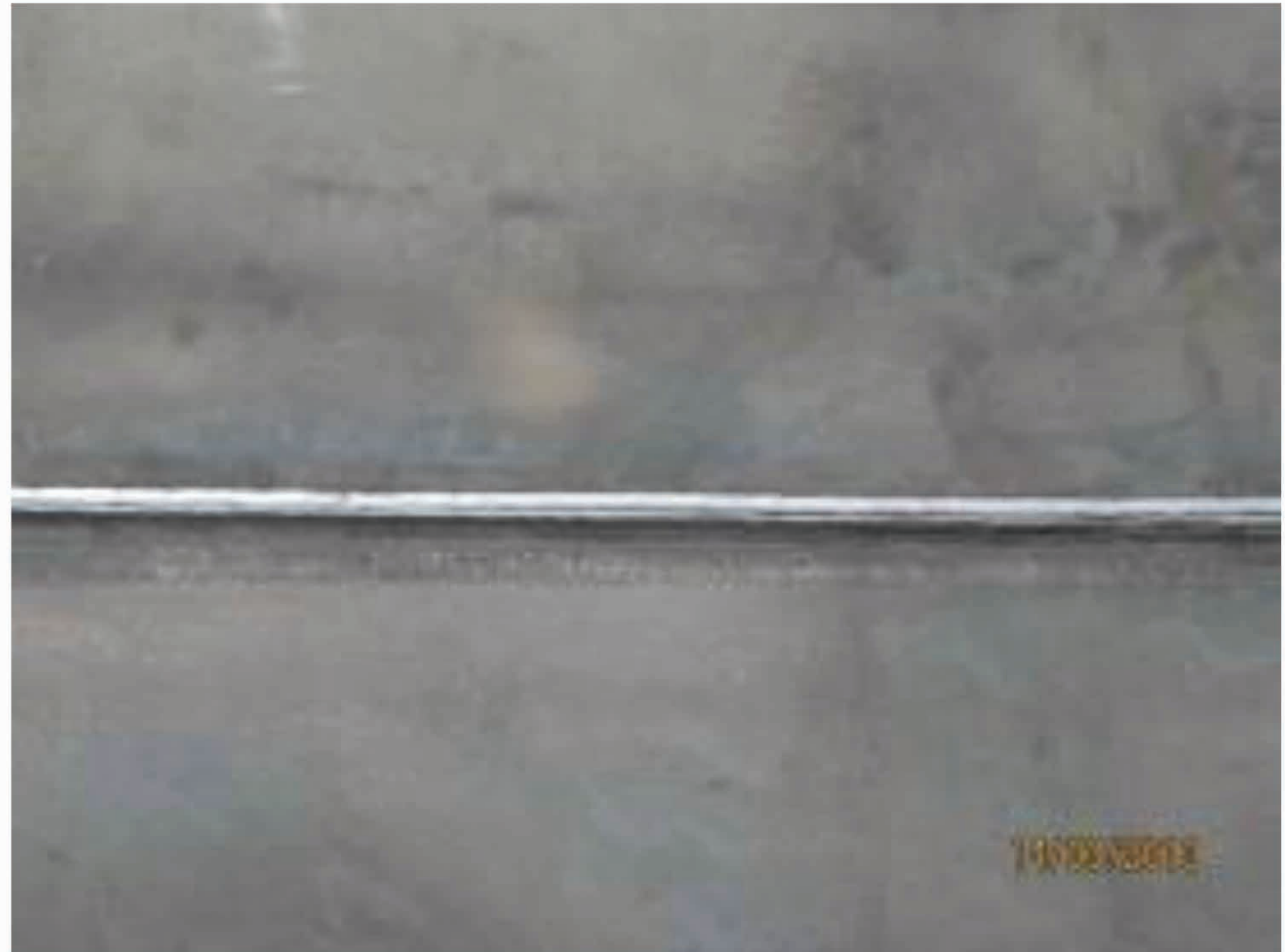
Vertical Seam & Girth Seam
