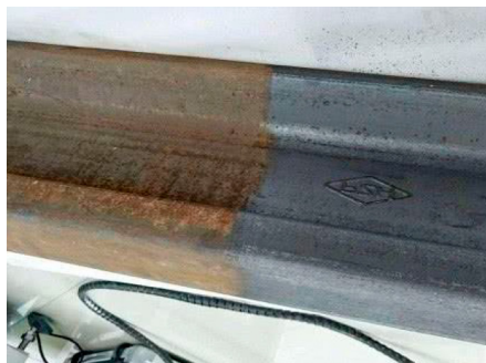
High-Speed Railway Track Rust Cleaning
